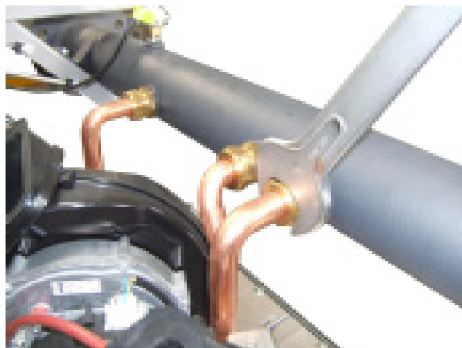
- Take out the gas fittings from the gas manifold with a 36 mm flat key.
